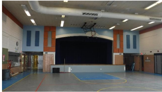
The recently completed stage at Schofield Elementary included a new stage curtain, acoustic panels, and lighting.
