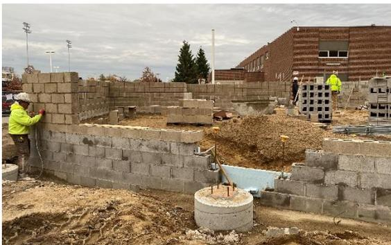
Foundations are in place and wall construction is underway at the new Fitzgerald High School Weight Room Addition.
